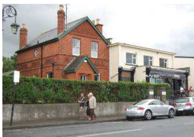
Fig 53. the gable fronted red brick building.
