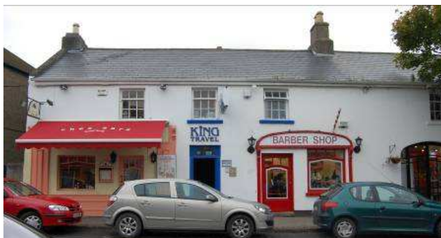
Fig 16. Building at intersection with Strand Street with historic display windows
