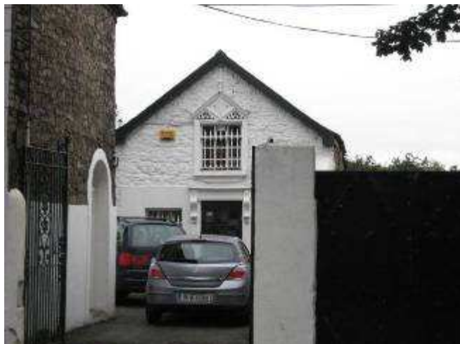
Fig 42. Outbuilding visible from New Street
