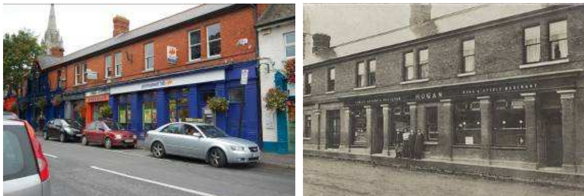
Fig 35. A new and old photograph of the red-brick terrace on the northern side of the Dublin Road approaching The Diamond
