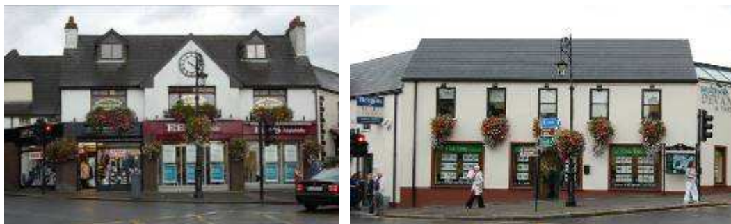
Fig 37. The south western and south eastern buildings
