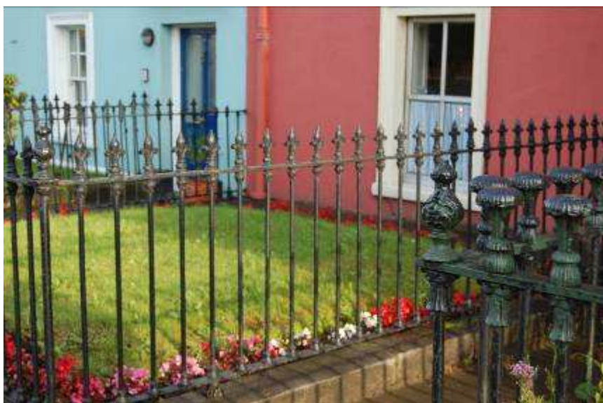
Fig 13. Railings along Castle Terrace
