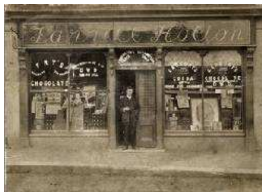
Fig 50. Historic view of same shop before subdivision
