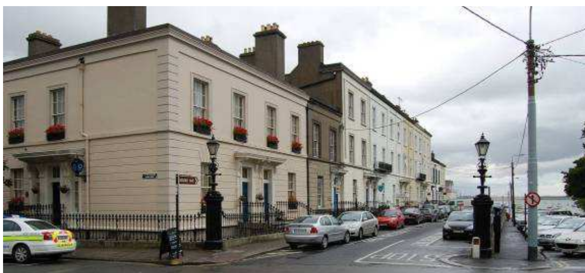
Fig 59. View of James' Terrace looking north
