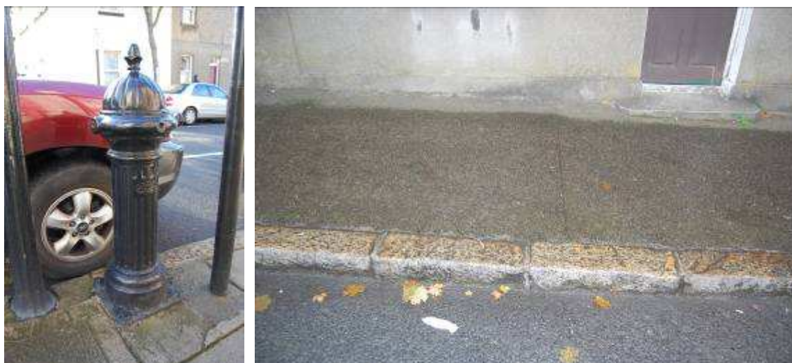
Fig 14. Water pump on Old Street and Fig 15. footpath and granite kerb on Old Street
