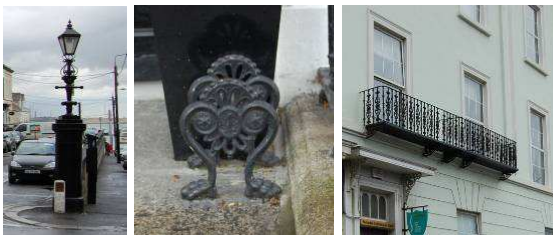
Fig 62. Attractive lamp standard at entrance to James' Terrace, not visible in historic photograph
