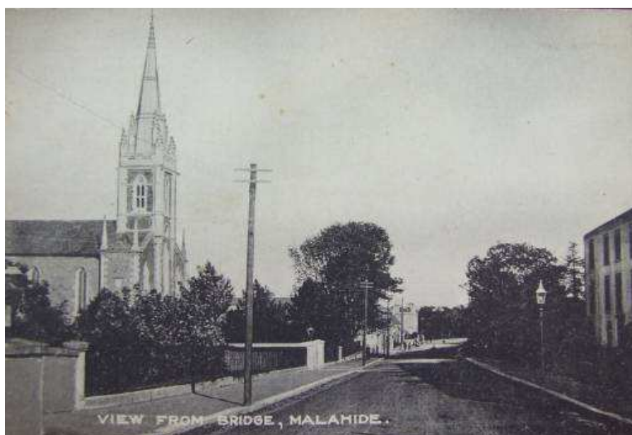
Fig 26. Historic view of the Dublin Road
